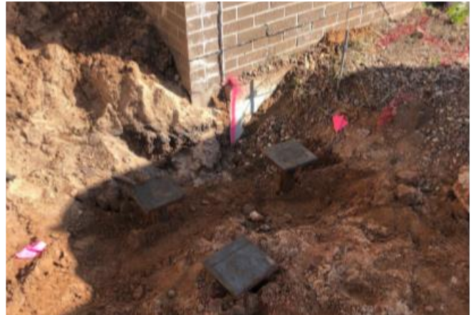
Helical Piers Installed - Fitness Center
