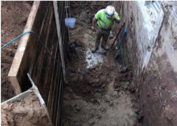
Retaining Wall – Fitness Center
