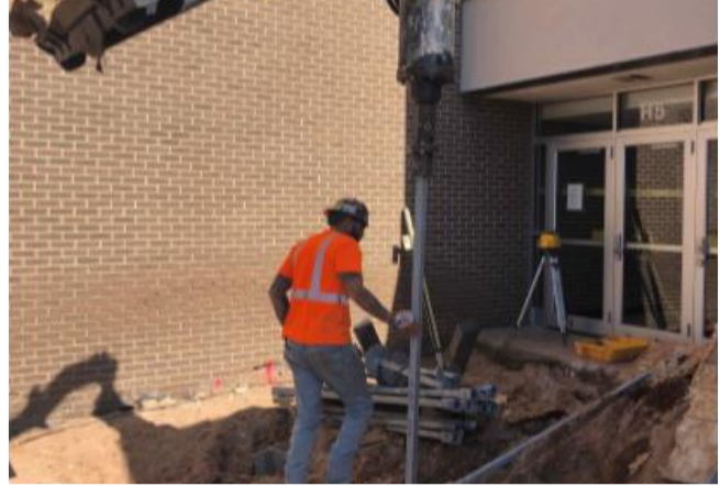
Helical Piers being installed – Fitness Center
